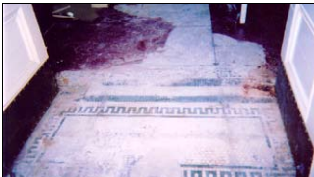
The Yorkville tile floor as uncovered during the May 2003 Retrofit.
